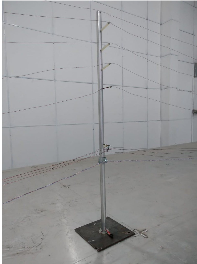
Fig. 32. Tower and line conductors (BATISTA MORAES et al., 2022).
