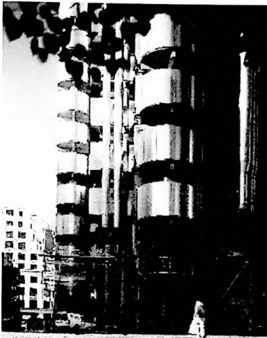
Lloyd's Building (1979-1986) Richard Rogers Fonte: Architectural Review, 1986, p.54
