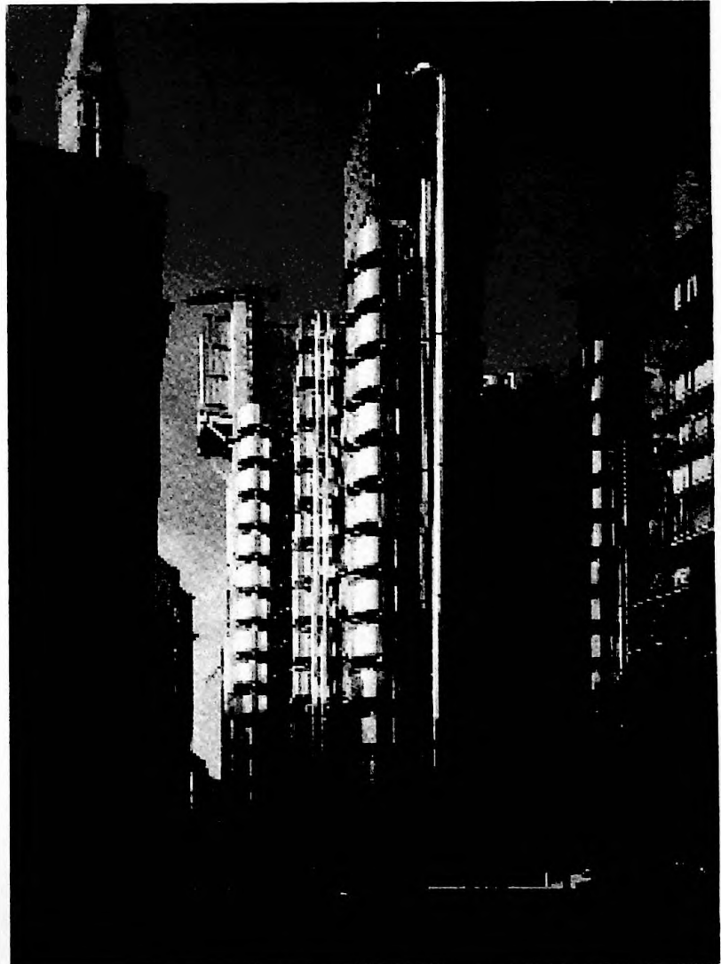
Lloyd's Building (1979-1986) Richard Rogers Fonte: Architectural Review, 1986, p.47
