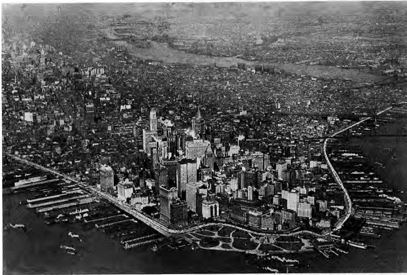
AIR VIEW OF SOUTHERN MANHATTAN, SHOWING RAISED WATERFRONT BOULEVARD PROPOSED BY NELSON P. LEWIS IN 1922
