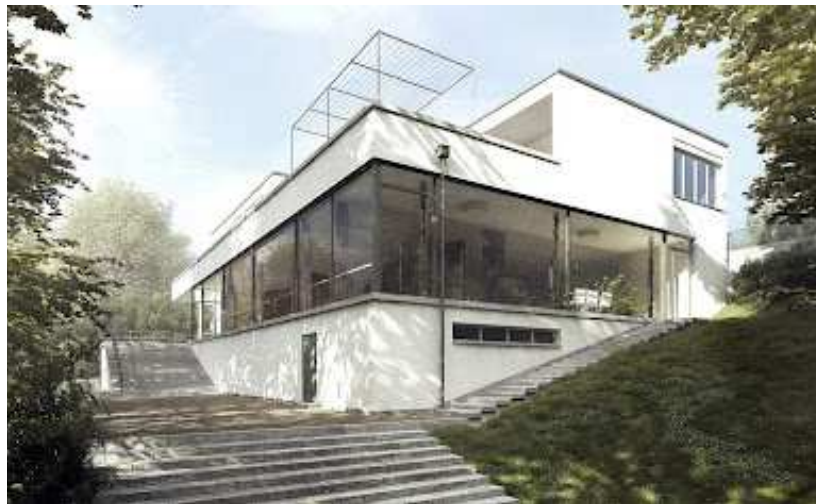
Fig. 24 Vista Lateral Casa TUGENDHAT Mies van der Rohe Fonte: http://pc.blogspot.com/2008/01/tugendhat-house-mies-van-der-rohe.html
