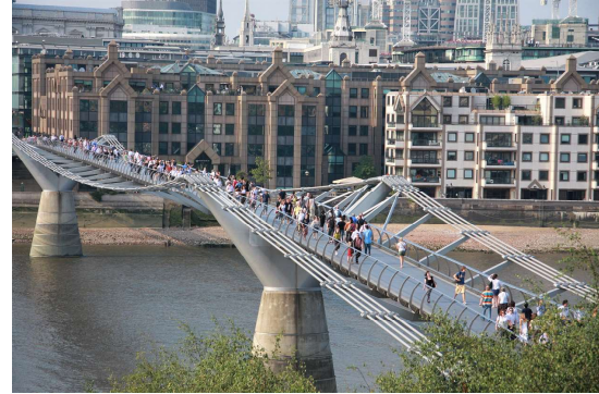
Figure 19: London's Millennium Bridge (60)
